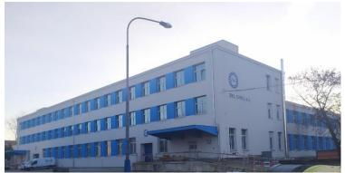
The reconstruction of building 32 and its modernization were designed for the entire building with the aim of reducing the carbon footprint. The newly created spaces were equipped with triple-glazed windows, and the floor was reinforced to withstand higher loads. A central hot water heating system was
